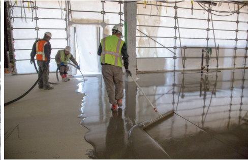
Floor Seal Technology technicians use PowerPump to apply the concrete moisture emission control and substrate leveling system.
